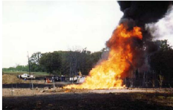
Figure 1-1: Post explosion flare-off of leaking gas from a burst pipeline. The burst was later attributed to corrosion weakened walls of the pipe. 2
