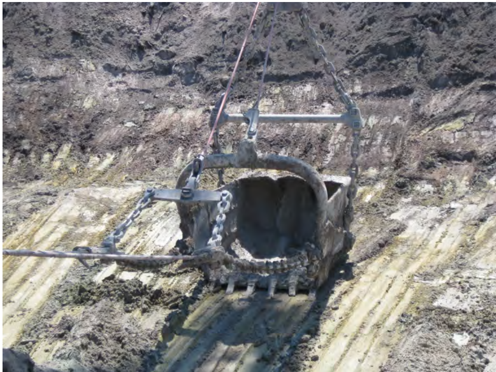
Figure 2-4. Photograph of bucket attached to the dragline used to displace the phosphate matrix (photograph by Mark Orazem, used with permission).
